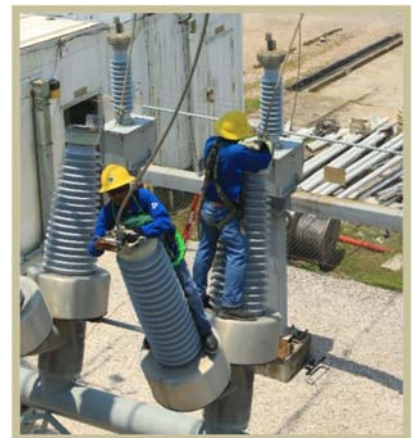
Maintenance of Magazine Rd Substation
