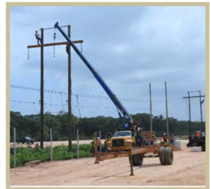
Relocation of transmission structures on Lake Independence Boulevard
