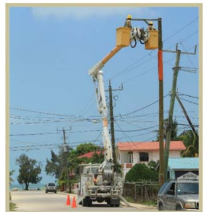
Upgrade of high voltage power lines
