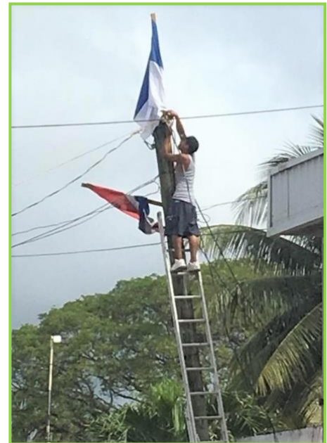
Man endangering his life by installing a flag on a utility pole and above power lines.
