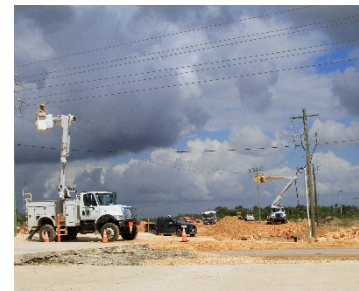
Relocation of poles
