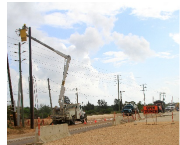
Relocation of power lines
